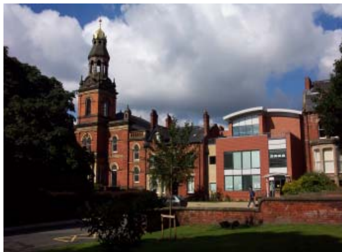
The new building of the School of Music, Leeds University; Brooks, Charles, Christina, Deborah, and Jennifer often met at the Wall by the awning on the right. Photo courtesy of Charles McGuire.
